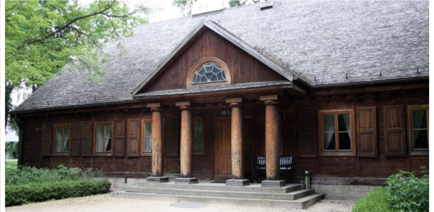
▼ Manor House in Radziejowice
