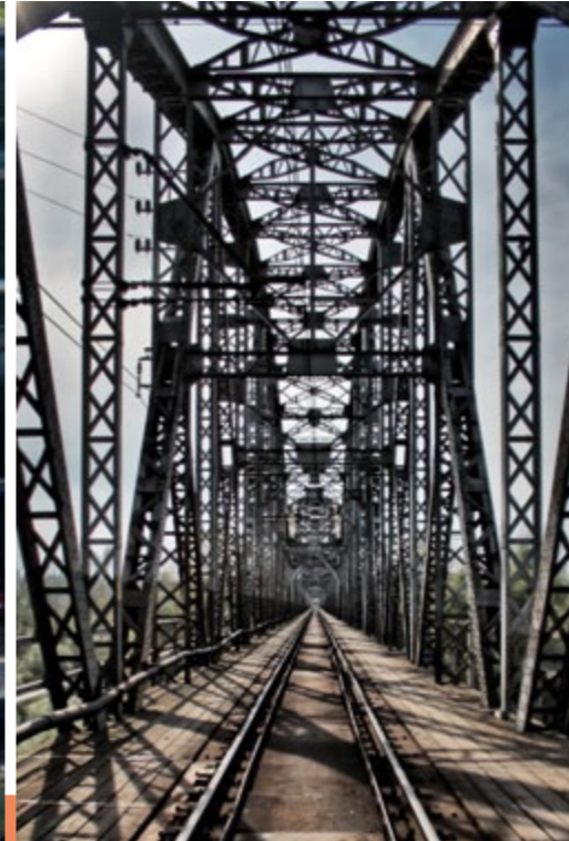
Bridge in Góra Kalwaria, Photo Marcin Salwa ▼
